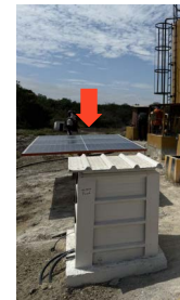
DUT-E S7 level sensor next to the main tank (left) DFM D S7 flow meter in the fuel line (center) Solar panel powering the CANUp gateway (right)
